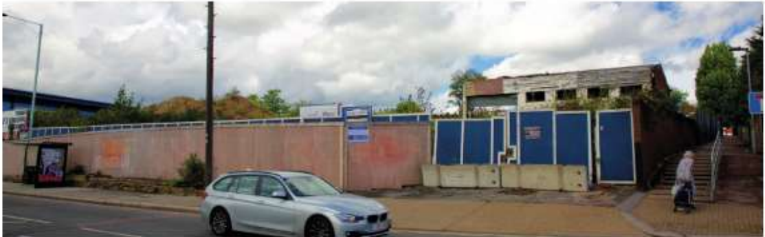
VIEW OF EAST ACCESS POINT
