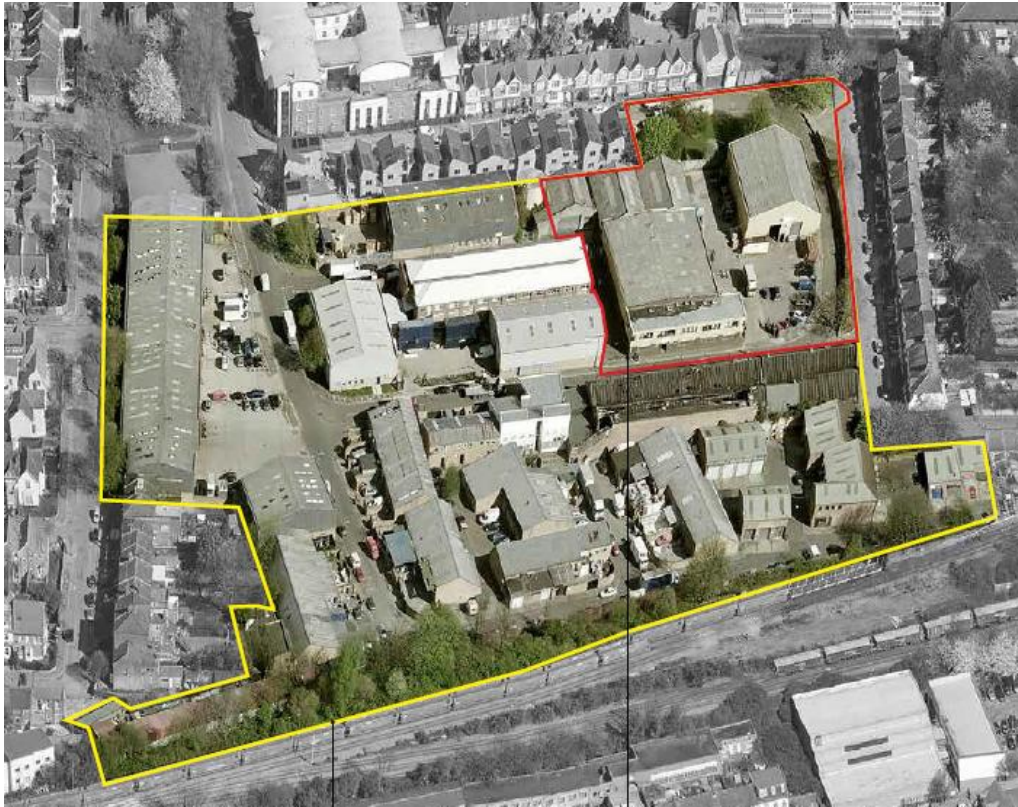
Image 1.1 –Historic Aerial Image - Rangemoor Road/Enterprise Row Industrial Estate (outlined in yellow) and application site outlined in red (top right corner).
